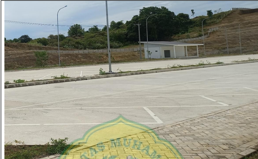
Gambar A.4.9 Bengkel Rest Area Km 37b
