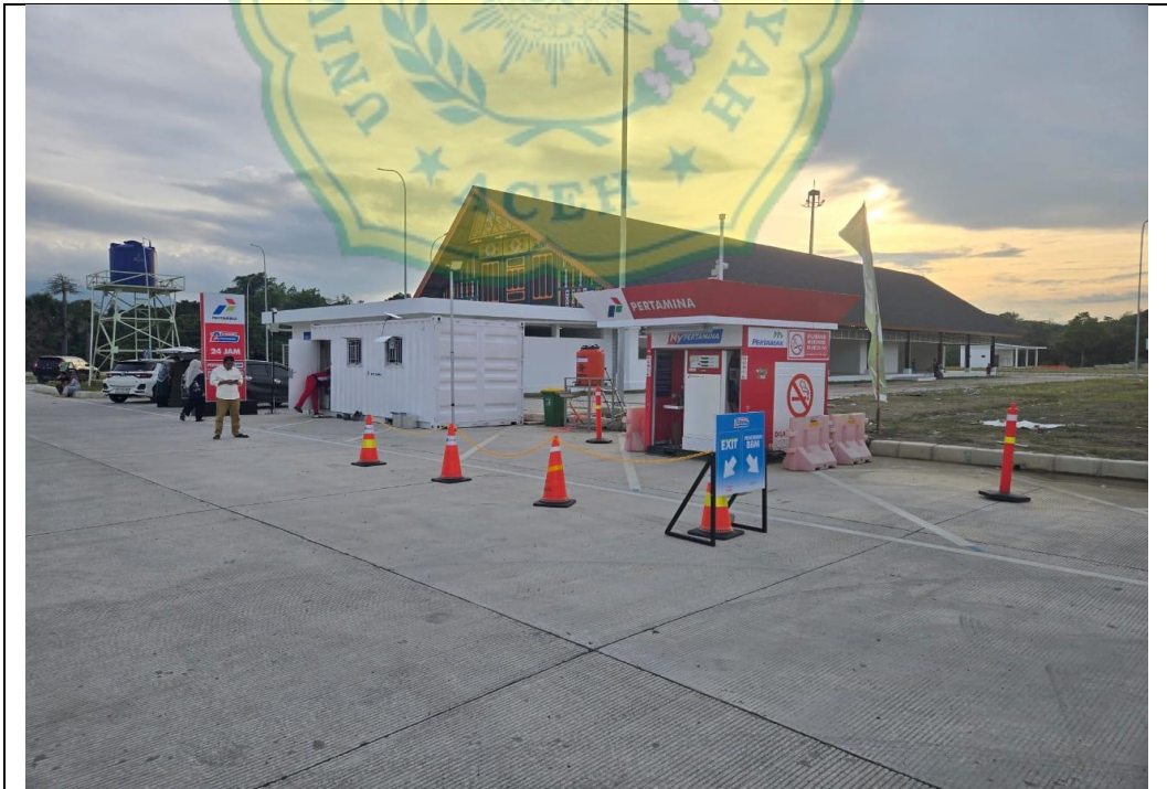
Gambar A.4.6 Fasilitas SPBU Modular Km 37b
