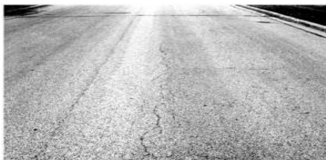
Gambar 2. 2 Retak Kulit Buaya ( Alligator Cracking ) Sumber : (ASTM D6433, 1995)
