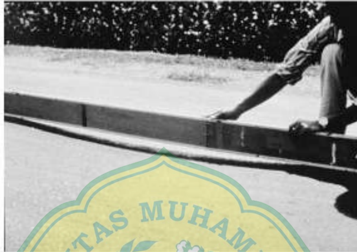
Gambar 2. 7 Amblas ( Depression ) Sumber : (ASTM D6433, 1995)
