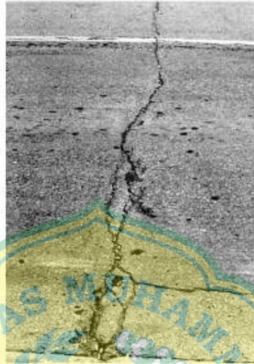
Gambar 2. 9 Retak Refreksi Sambung ( Join Reflection Cracking ) Sumber: (ASTM D6433, 1995)
