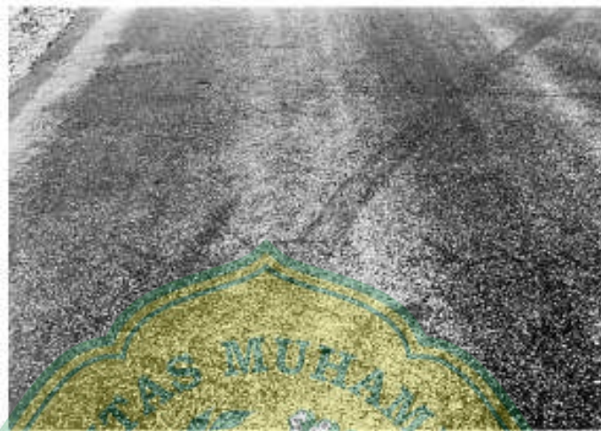
Gambar 2. 3 Kegemukan ( Bleeding ) Sumber : (ASTM D6433, 1995)
