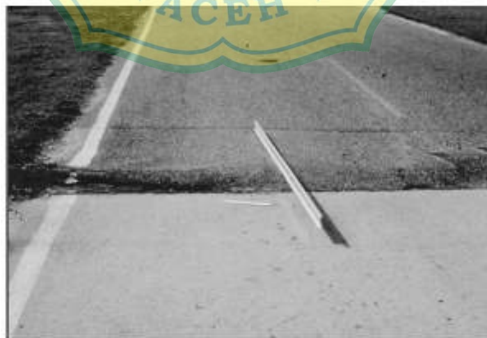
Gambar 2. 16 Sungkur ( Shoving ) Sumber : (ASTM D6433, 1995)
