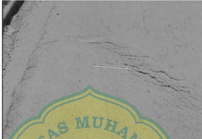
Gambar 2. 17 Retak Slip ( Slippage Cracking ) Sumber : (ASTM D6433, 1995)
