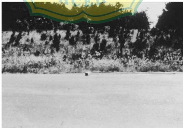
Gambar 2. 18 Mengembang (Swell) Sumber : (ASTM D6433, 1995)
