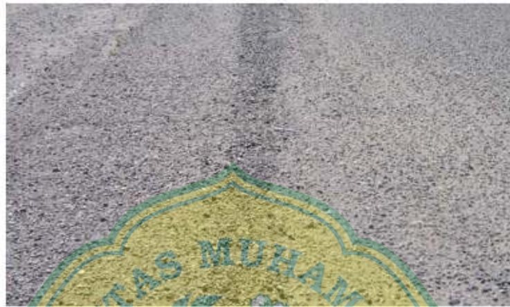
Gambar 2. 19 Pengelupasan dan Butiran Lepas ( Weathering and Raveling ) Sumber : (ASTM D6433, 1995)
