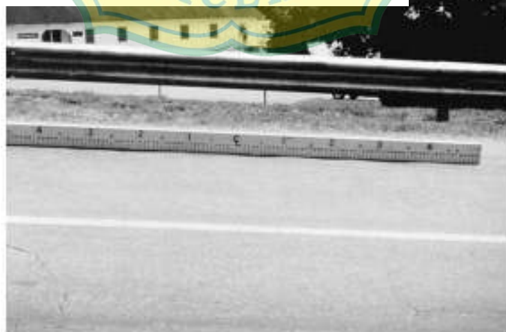
Gambar 2. 6 Keriting ( Corrugation ) Sumber : (ASTM D6433, 1995)
