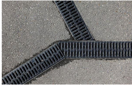
Gambar 4.12 Drainase Tertutup ( Sumber : https://www.google.com.jenisjenisdrainase )
