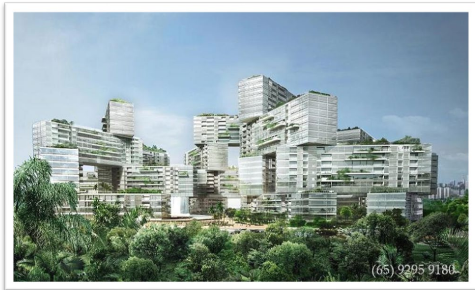
Gambar 2.15 : Apartemen The Interlace Condominium In Singapore
