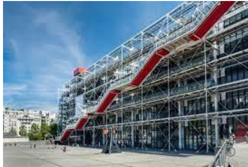
Gambar 3.1 Pompidou Centre, Paris
