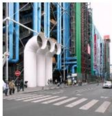
Gambar 3.4 Pompidou Centre, Paris
