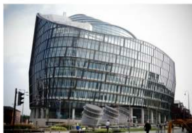
Gambar 5.14. Double Skin Façade (Sumber : www.modlar.com/foster-fasade )
