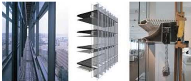
Gambar 4.16 Double Skin Facade (Sumber : http://www.controlyourbuilding.com/ )
