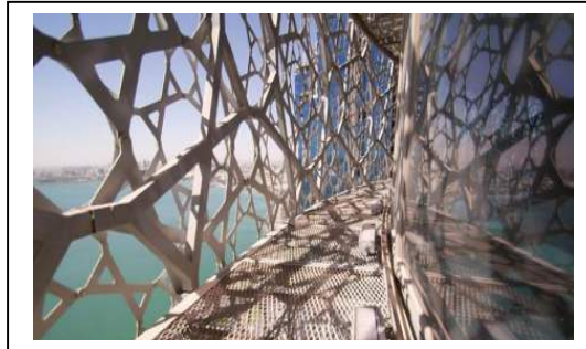
Gambar:5.21 Sistem secondary skin (Sumber :analisa 2020)
