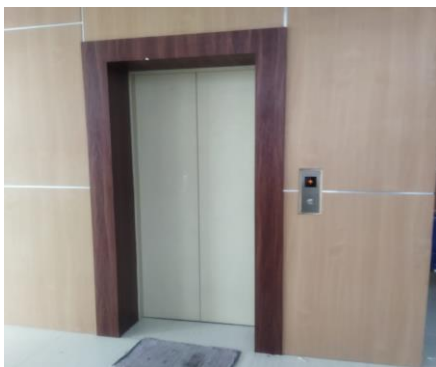
Gambar 2.9 Lift Sumber : Survey Lapangan, 2022
