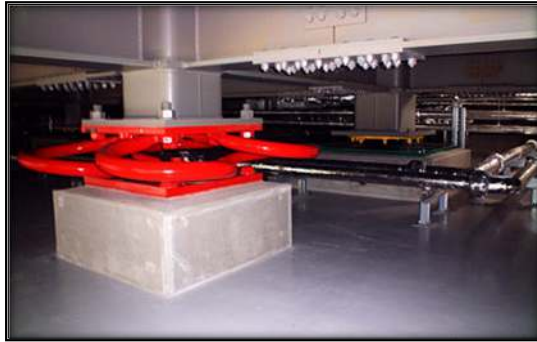
Gambar 5.7. Base Isolation System
