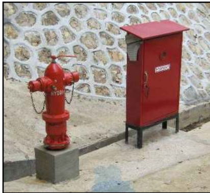
Gambar 5.16 Fire Hydrant (Sumber : Google Image, 2018)
