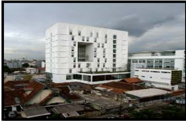
Gambar 2.19 : Morrissey Hotel (Sumber : Archdaily, 2022 )
