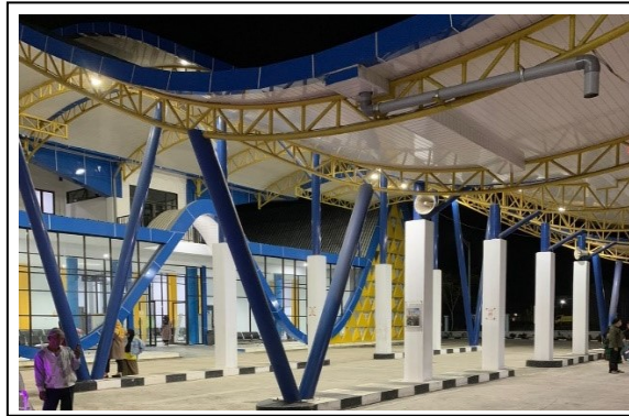
Gambar 5.21 Struktur Space Frame (Sumber: https://www.buildipedia.com ,2023)
