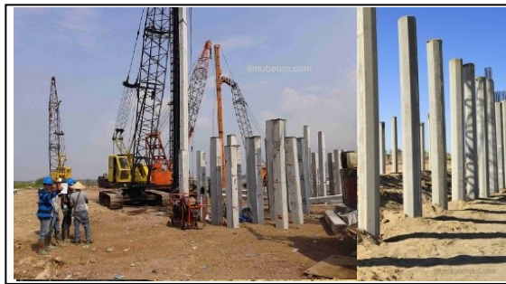
Gambar 5.19 Pondasi tiang pancang (Sumber: https://www.ilmubeton.com ,2023)
