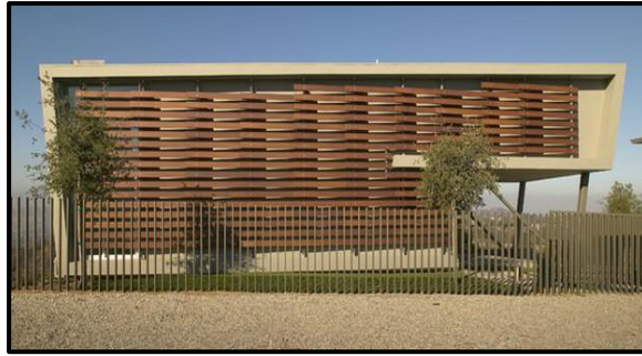
Gambar 3.8 Tampak Skyline Residence Sumber: www.arsitag.com
