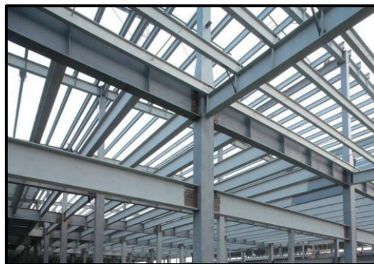
Gambar 5.12 Baja WF ( Wide Flange ) (Sumber: http://www.teknik-sipil.com , 2019)
