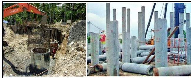
Gambar 5.8 Pondasi Sumuran (Sumber: https://www.ilmubeton.com , 2023)
