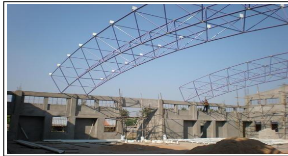
Gambar 5.10 Struktur Space Frame (Sumber: https://www.buildipedia.com , 2023)
